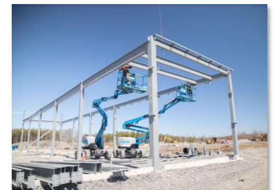
Construction of New Fiberglass Facility in Kingston, Ontario
